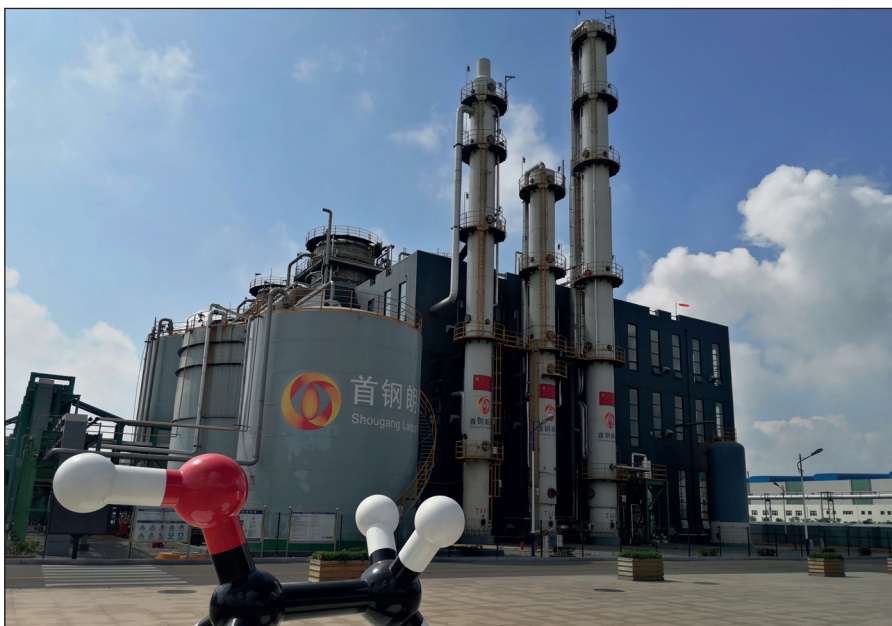
Above: Carbon dioxide for this project is captured from the steel-mill waste stream of China's Shougang Group Right: An essential part of the process is the bioreactor containing the brew of microbes
